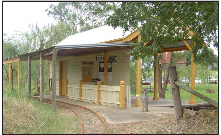
Kurrajong railway goods shed constructed 1926
