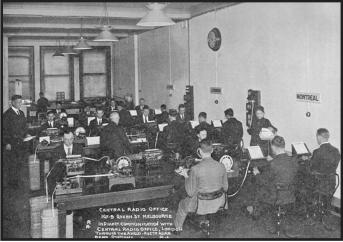
**CENTRAL RADIO OFFICE, QUEEN STREET, MELBOURNE.** Central Radio Office, Queen Street, Melbourne, where Beam Stations (50 miles away) are operated by distant control and messages are sent direct into the City of London. Other wireless services are also operated from this central control office.
