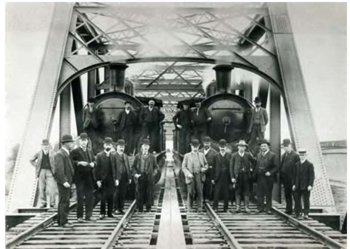
New Railway Bridge across the Nepean 1907 (Testing day, before Official Opening) Image: Glenbrook Historical Society
