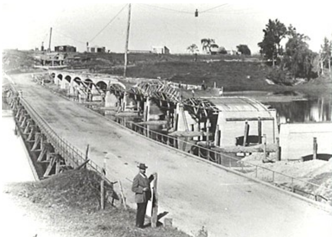
The new Richmond Bridge in 1904 under construction over the Hawkesbury River. The gentleman is standing at the edge of the old bridge crossing.
