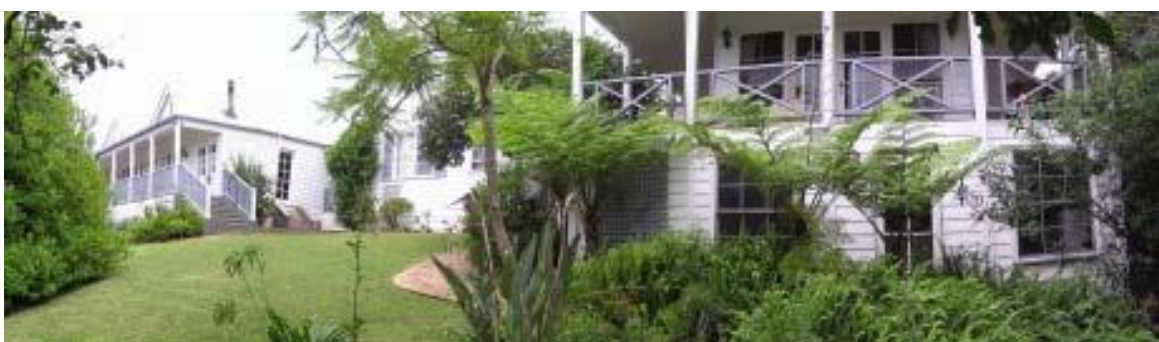
Below: The rear of Loxley today, showing some of the extensive gardens, and showing how the redevelopment has kept in good harmony with the style of the original building. (Photo by Greg Upton).
