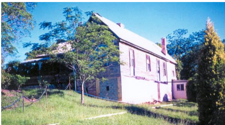
The western side of "Plynlimmon" showing its neglected state in 1988. Image 190303
