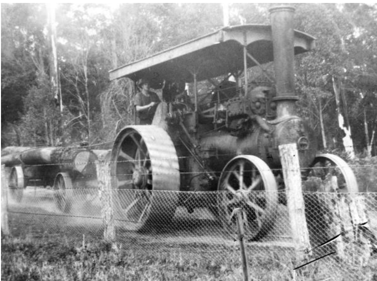
The steam tractor (traction engine) pulls the timber jinker loaded with logs near Hobby Bros Sawmill, Bells Line of Road, Kurrajong Heights, not far from the Bowling Club. c. 1920s Image 034901
